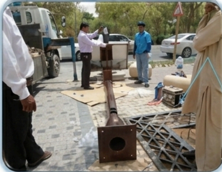
Installation of Street Light Pole
