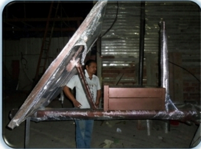
Assembling of Pole
